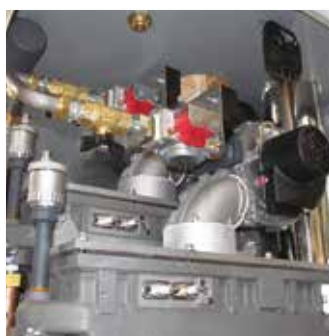
Group of: fan, modulating gas valve, premix burner
